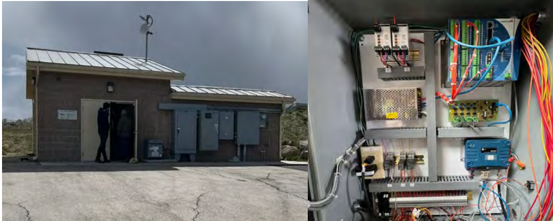
Figure A-20: Zone 3 0.5 MG Tank
