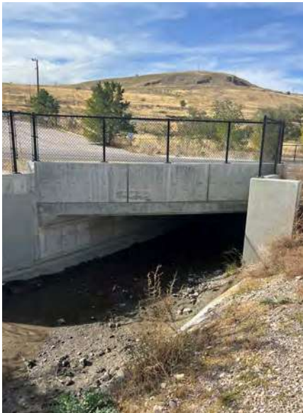
A canal crossing on the route.
