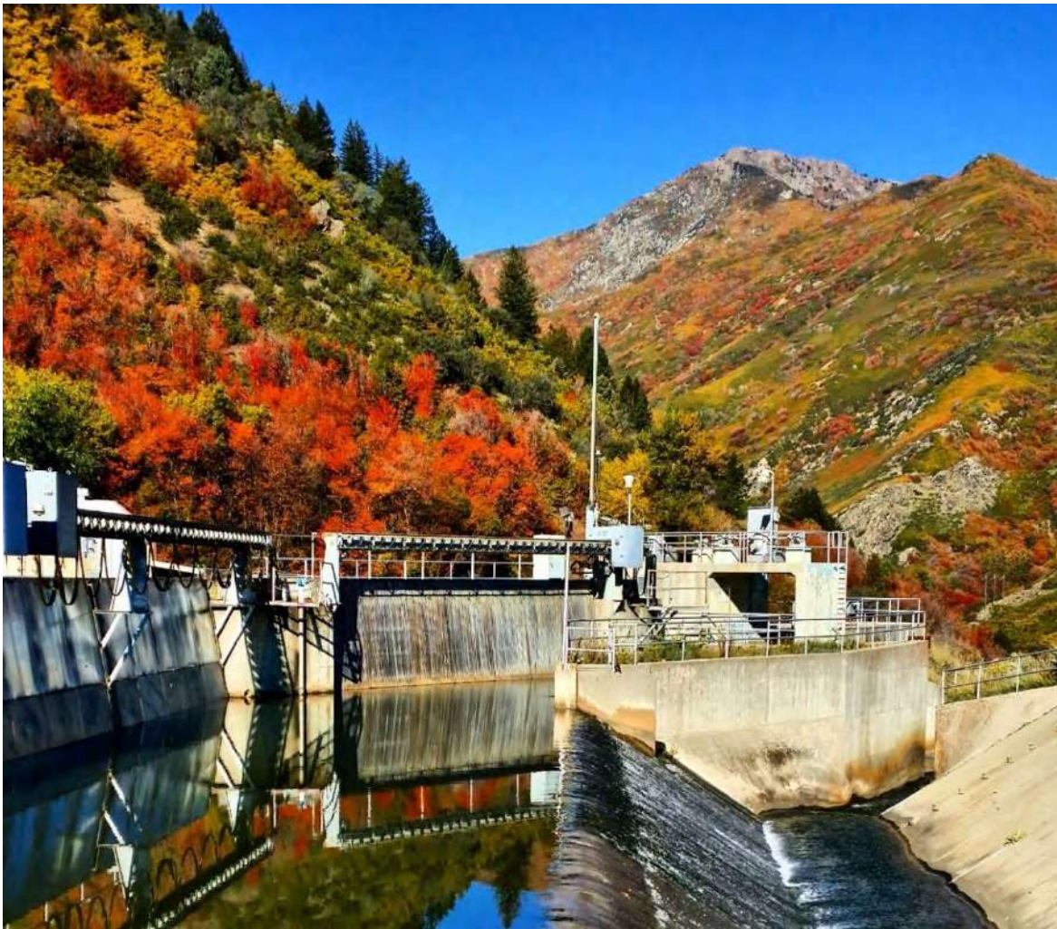
Diversion structure in Weber Basin
