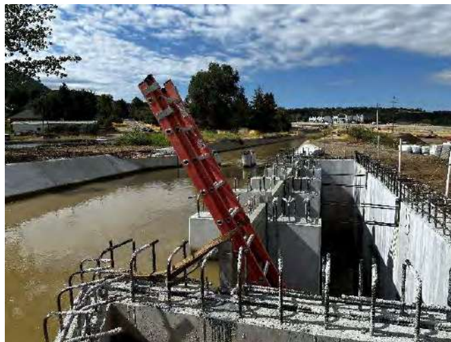
Aqueduct construction work in Weber Basin
