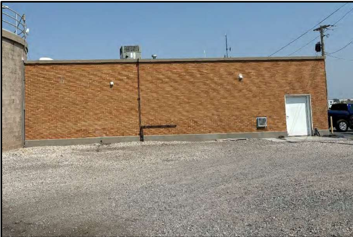
Photo 2 - Operations Building West Elevation
