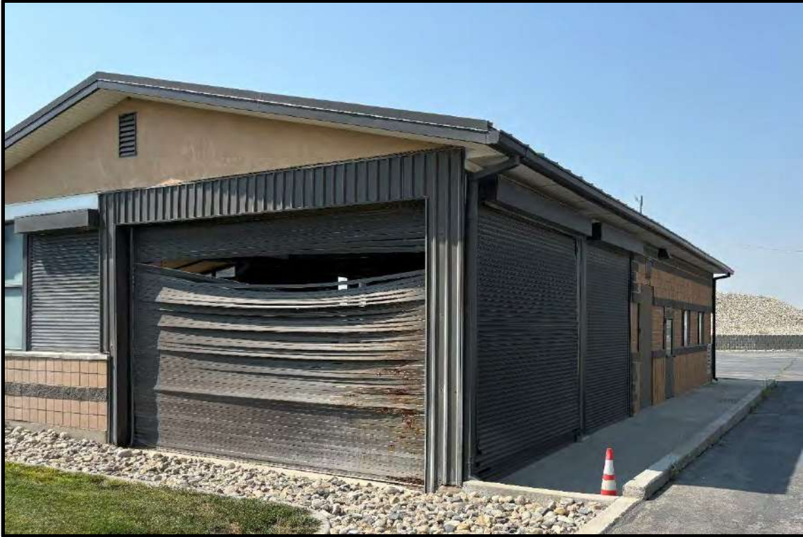
Photo 11 – West Headworks (Location for Alternative 2)
