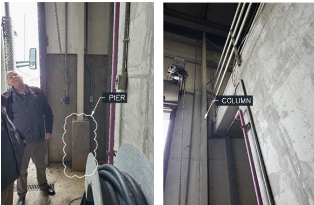
Picture 13: Concrete column pier
